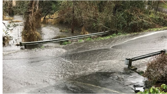
Figure 10 - 8th Ave NE flooded by winter rain. Image: submitted via survey
